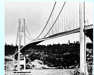
Tacoma Narrows Bridge, 7. Nov. 1940.
